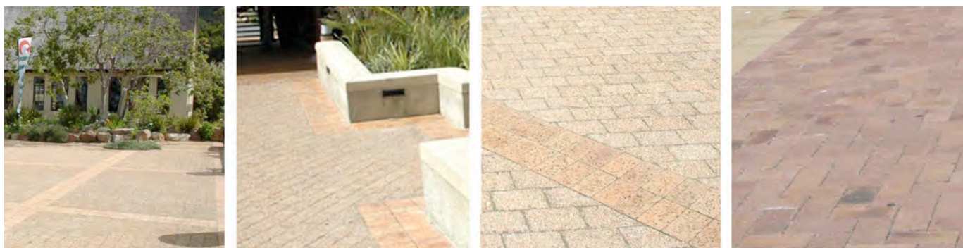
Kirstenbosch Gardens - Autumn blend exposed aggregate paver with a smooth brick double band edge. Variations of this natural colour would be appropriate for hard landscaped areas within the residential fabric.
